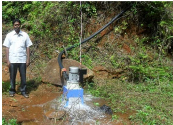
Figure 7-4: Microhydro power facility (Source: Home Power [9])
